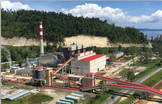
Captive power plant project in Brazil, which has been combined to the grid
