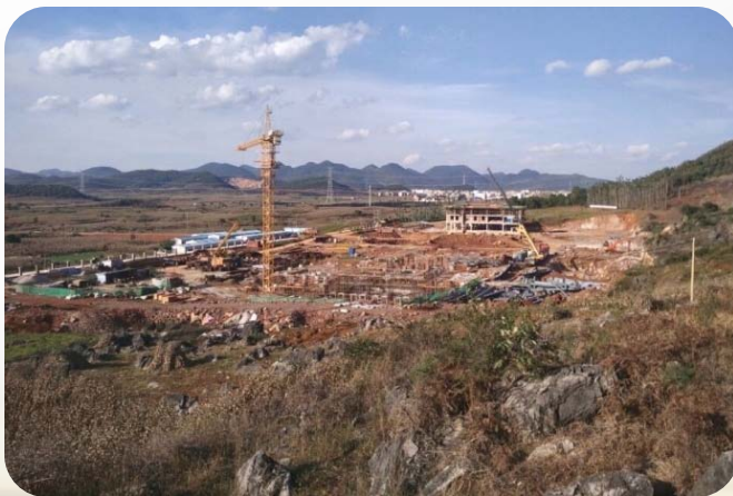
Grate furnace waste power generation project under construction in Yanshan.
