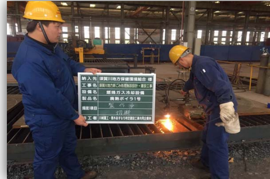
Officially start the boiler manufacturing work for Sukagawa project in Japan.
