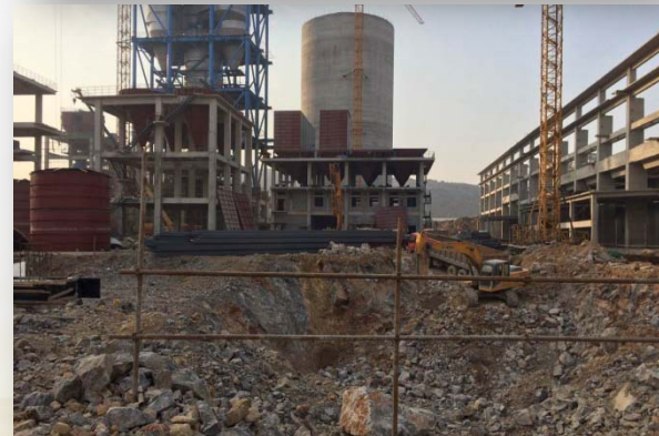
Solid waste disposal projects under construction in Wuhu, Huaibei.
