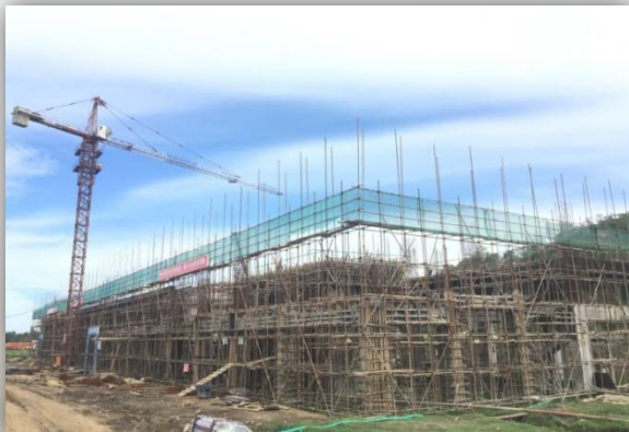
North Celebes Project under construction in Indonesia.
