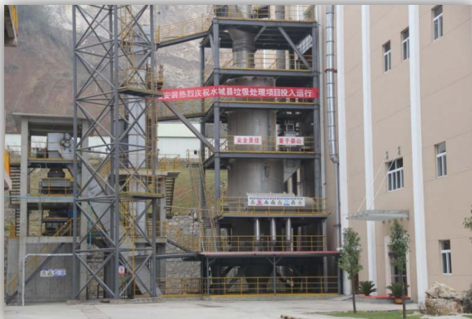
Shuicheng Project in Guizhou was completed and put into operation.
